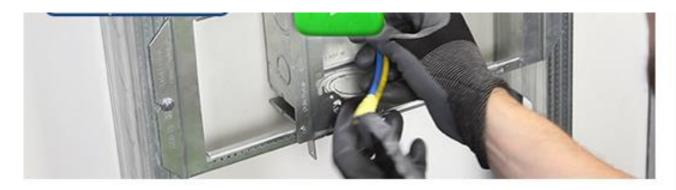
Want a **complete solution** to rough-in datacom boxes? Order the <u>Pre-assembled Simple Support Bracket with 5" Square Box</u>. Take the SSB-T5B-200 out of the package, zip it between studs, and you're done! Includes <u>UMA-LVBS</u> (see #3) -- <u>SSB-T5</u> -- <u>T5B-200</u> -- <u>T5R</u> -- and pre-installed #8-32 screws, ready to take a 4" ring!
